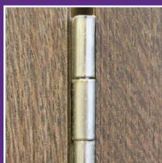
Continuous piano hinge
